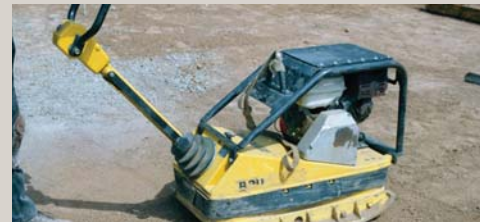
Compaction should be performed when the moisture content of the soil is slightly above its optimum.
