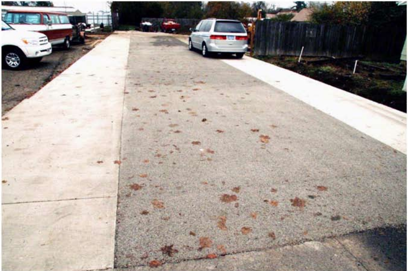
Adell St, OR, pervious pavement
