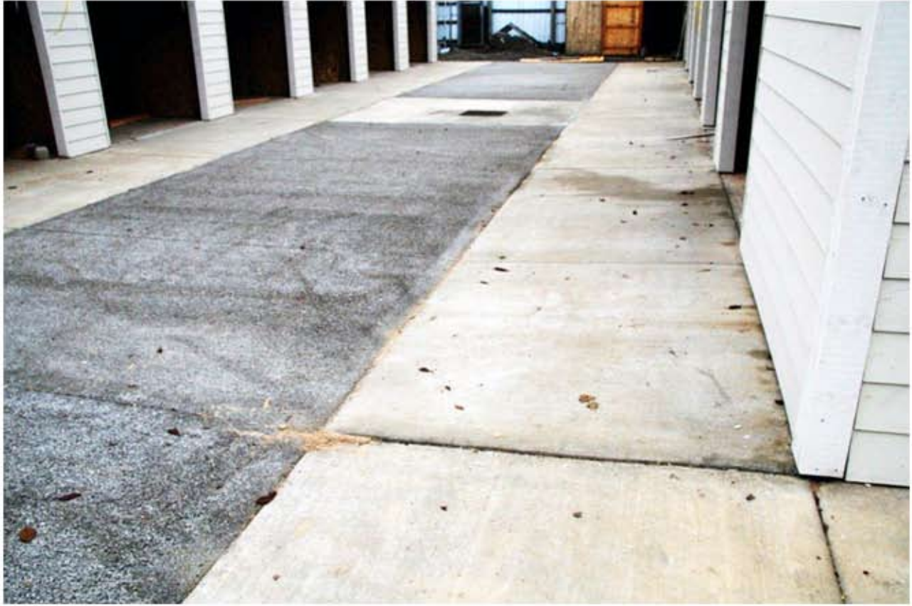
Adell St, OR, under construction
