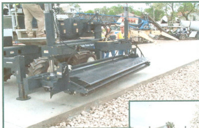
Concrete was placed using a pervious head on Somero's SXP screed.
