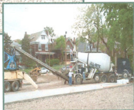
Pervious concrete was placed using a telebelt.
