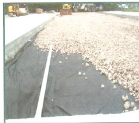
Under-slab drainage.
